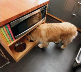
Clever island assembly. The butcher-block island top was made by butting together two counter-depth pieces. The base is made from a pair of Ikea drawer units. Custom shelves at one end hold the microwave and bowls for the dog's food and water.
