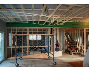
Bones of the wave. The framers used a plywood template to position strapping on the ceiling to support 16-ft. lengths of drywall. The result was an undulating ceiling that flows over the bright, airy kitchen. All appliances were salvage finds and kept costs low.
