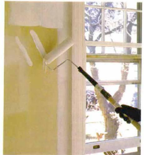
**The end of the ropes.** Ropes, or heavy lines of paint, show up when there is too much paint on the outer edges of the pad. Running the edge of the roller on the wall squeezes out the excess paint.
