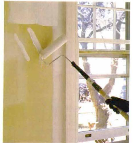
**The end of the ropes.** Ropes, or heavy lines of paint, show up when there is too much paint on the outer edges of the pad. Running the edge of the roller on the wall squeezes out the excess paint.
