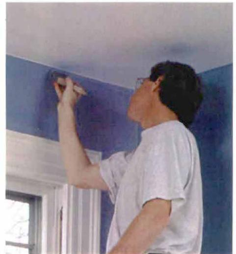
**Final finicky cut in.** The final cut in is the most crucial to make sure the line between ceiling paint and wall paint is perfectly straight.
