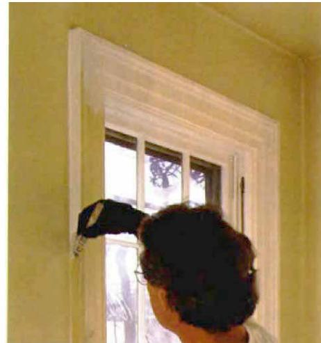
**Caulk before you paint.** Before the walls or trim is painted, a bead of paintable caulk is applied to fill the gap between the trim and the walls.
