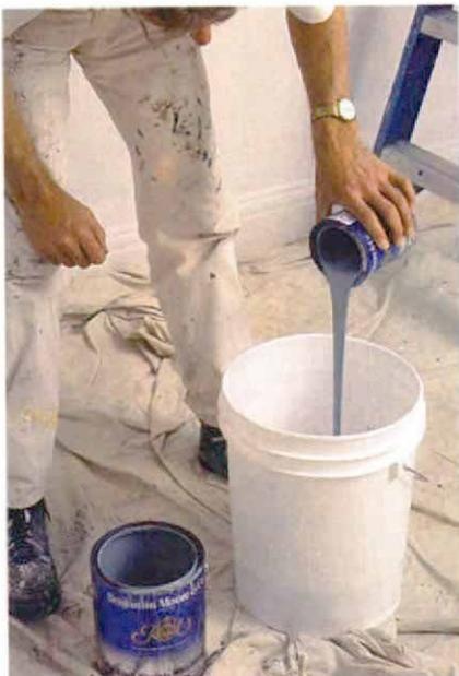
**Blend all the finish paint together.** Custom-mixed paint can vary in color from can to can, so all the paint is mixed together in a 5-gal. pail before it goes on the walls.
