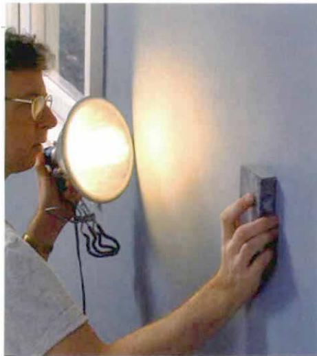
**Smoothing the walls between coats.** A work light helps to find any lumps or debris in the first coat. A light sanding smooths everything out.
