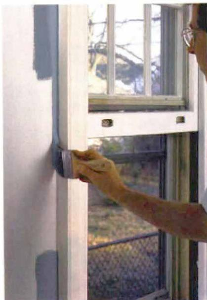
**You're getting paint on the trim.** Overlapping paint between adjacent surfaces continues as the wall paint is extended onto the trim slightly. The finish paint on the trim will create the final line.
