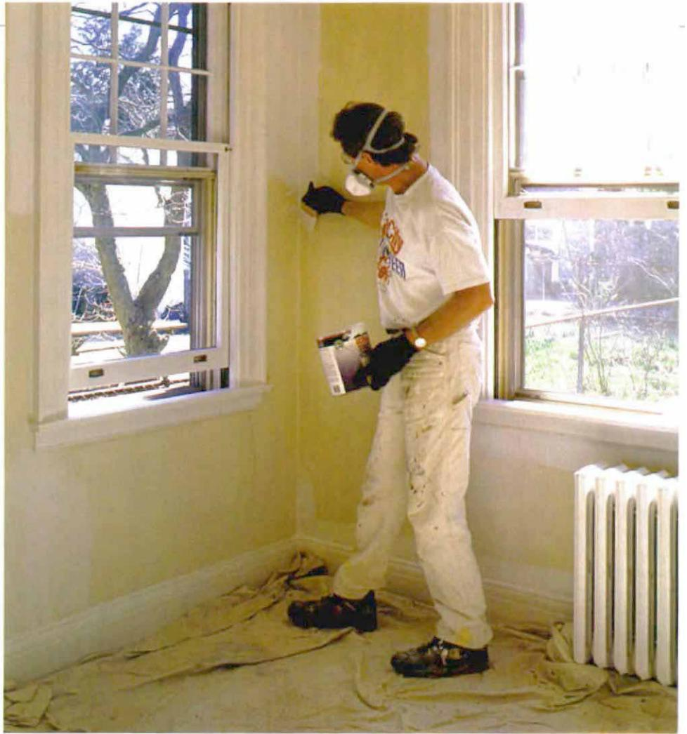
**Cutting in from the floor.** The author first cuts in the upper part of the room from a ladder, then works his way around the room, standing on the floor and cutting in.
