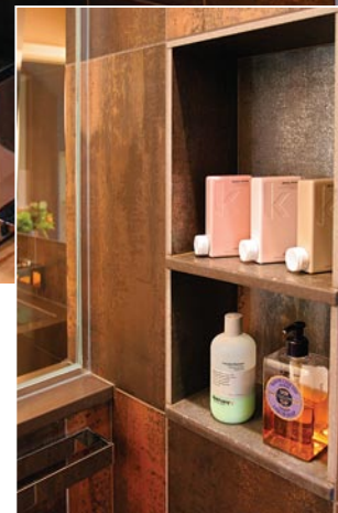
Tile with style. The large shower is accentuated with vertical 12-in. by 24-in. wall tile and a mosaic-tile floor. Cast-concrete sills, shelves, and threshold complement the vanity sinks. Photo taken at C on floor plan.
