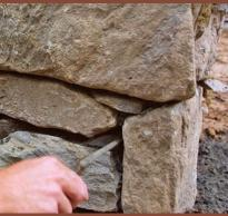
Rake out the semidry mortar. After a few hours, the mortar is dry enough to remove all that is visible. Use a pointing trowel and go deep. There should be no visible mortar in a dry-stack veneer wall.
