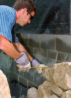
**Keep the rocks plumb.** Regardless of how thick the rocks are, the faces should be in the same plane. If the foundation wall is plumb, you can measure to the face of the rocks consistently.
