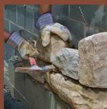
Use shims to set the stones more securely. The rock-fragment shims can be used in one of two ways: either as temporary shims until the mortar sets up or as permanent plugs to fill gaps between stones, giving a tighter appearance.
