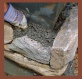
Pack mortar behind the stones. Mortar holds the stone in place, and wall ties embedded into the mortar tie the stone veneer to the block wall. Lay a mortar bed on top of each stone course for the next course.
