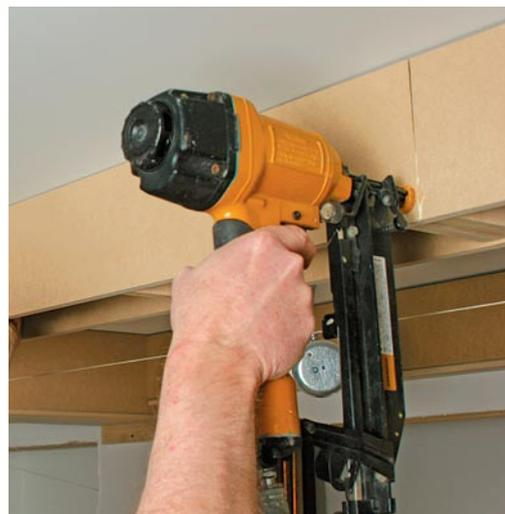
**Beveled joints make long runs look seamless.** Once the long piece is nailed, I scribe and install the short piece. I tune the beveled and butt ends of this piece as needed for the best fit. Gaps at the ceiling will be covered by bed molding.
