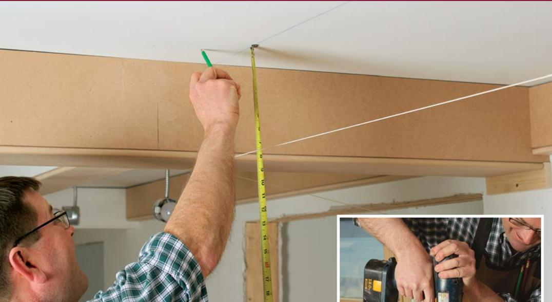
**Make the beam bottoms level.** I build the deep beams first, then run a stringline between them as a reference for level. Measuring down from the ceiling enables me to find the low points. Next, I cut all the ribs for the blocking using this measurement, taking into account the cleat and beam-bottom thicknesses, and the beam's height. I then glue, nail, and screw the ribs to the cleat every 16 in. on center. I use two 2-in. screws per rib.
