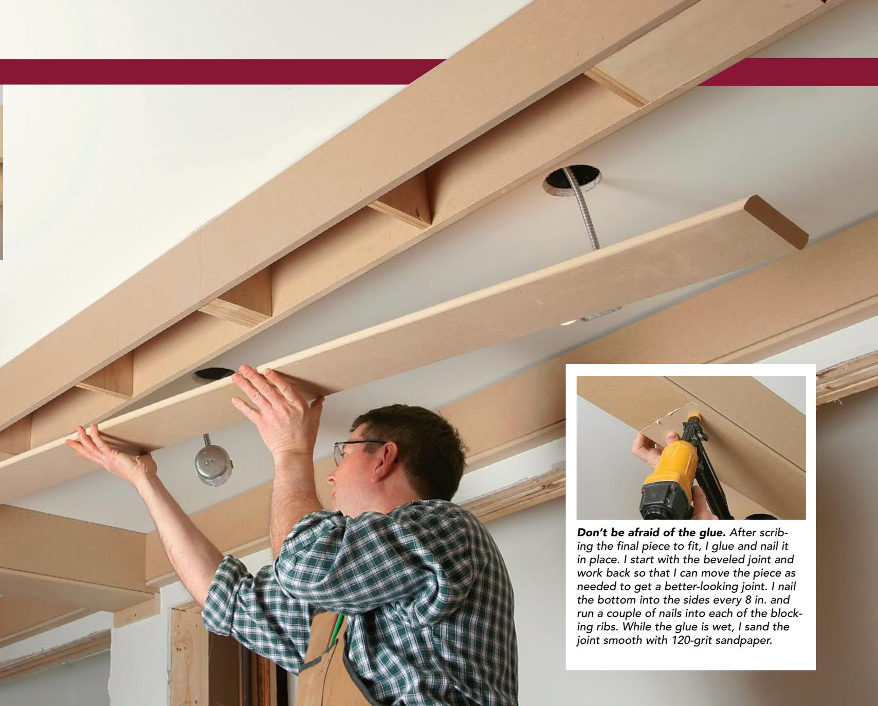
**Don't be afraid of the glue.** After scribing the final piece to fit, I glue and nail it in place. I start with the beveled joint and work back so that I can move the piece as needed to get a better-looking joint. I nail the bottom into the sides every 8 in. and run a couple of nails into each of the blocking ribs. While the glue is wet, I sand the joint smooth with 120-grit sandpaper.
