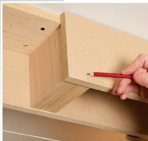
**Cleats and ribs offer plenty of nailing options.** Although temperature and seasonal changes don't affect MDF much, I still like to nail it well. I apply glue to the blocking assembly and run two or three 2-in. finish nails into each rib, as well as two nails into the cleat between each rib. To save time, I eyeball the short-point cut for the beveled joint instead of measuring.
