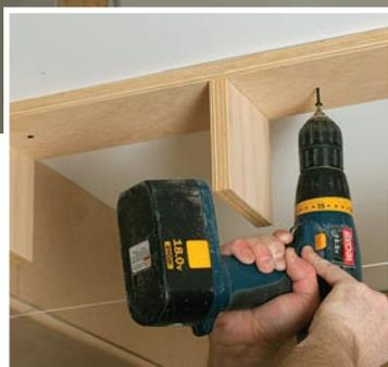
**Long runs go up in sections.** I build and install a full 8-ft. section first, then build the remaining section to fit. The doubled-up ribs at adjoining ends become the backing for the side's joints. Each blocking section is glued to the ceiling with construction adhesive, then screwed into ceiling joists and furring strips that I installed beforehand. For each joist, I use two screws long enough so that at least 1 in. sinks into the joists or furring.
