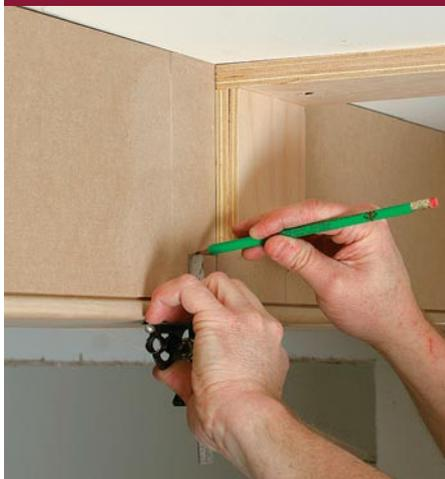
**Intersecting beams provide a good reference.** Deep beams are level along their bottom edges, so the reveal between them and the shallower beams should be uniform. This helps to fool the eye into thinking that the ceiling is level. I mark the low point of the sides on the deep beams using a combination square.
