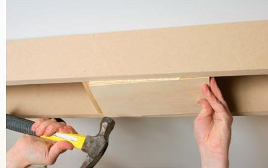
**Add blocking no matter where this joint lands.** In most finish-carpentry jobs, staggering the joints is a good rule to follow. When running the beam bottoms, I start with a full 8-ft. run as I did with the blocking assembly and sides. But I make sure the joint lands on the other end of the beam. Even if the joint falls on or near a rib, I install extra blocking for a larger nailing surface.
