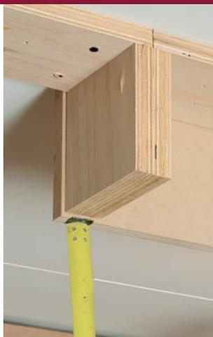
**Test-fits reduce the proliferation of four-letter words.** I rip the sides based on the ceiling's low point. With the side piece in place, I then measure up from the stringline to make sure the board is the right width to maintain a straight, level run. When I'm working alone, a cleat nailed to the cross beam provides a helping hand.
