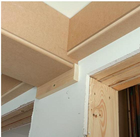
**Transitions and terminations require some forethought.** In low ceilings when the beam terminates into door or window casing, I hold the beam bottom back using a scrap piece of trim. When I install the trim, I remove the block and slide the casing in its place. I also run beams around the perimeter of the room. Using only part of the beam width implies their structural function, and provides a way of tying in door and window casing as well as built-in cabinetry throughout the room.
