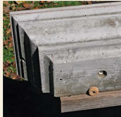
Recessed for screw head. Prying out the cork makes room for the heads of the screws. The pilasters conceal these connections.
