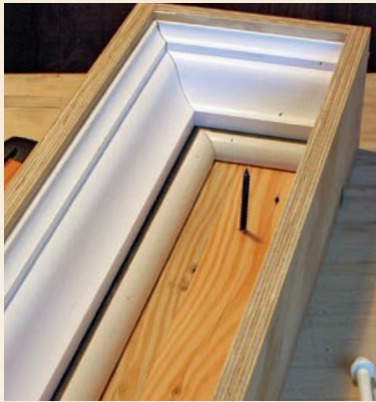
Inside the mantel form. A 1/4-in.-dia. screw at each end of the form positions sleeves cut from 3/8-in.-O.D. plastic water-supply tubing. Screws that run through these sleeves hang the mantel from the chimney framing. A section cut from a wine cork creates a knockout for the screw head and its washer.
