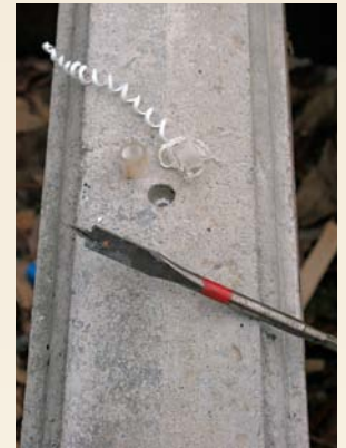
Holes for pilaster screw caps. A short knockout of 1/2-in.-O.D. plastic tubing pressed onto the 3/8-in.-O.D. sleeves creates a cavity for the screw heads. Running a 7/16-in. spade bit into both the knockout and the sleeve hollows out the recess.
