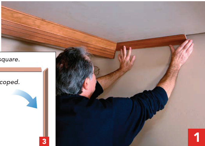
1 Set the spring angle. Tack the first piece of crown in place at the right using a coped scrap to set the correct spring angle.
