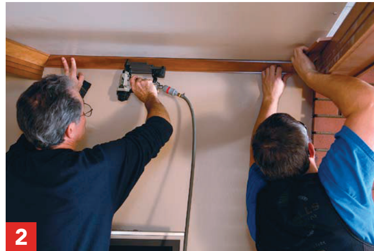
2 Repeat on the second piece. Register the left-hand cope against the first piece, set the angle of the right-hand side, and nail in place.
