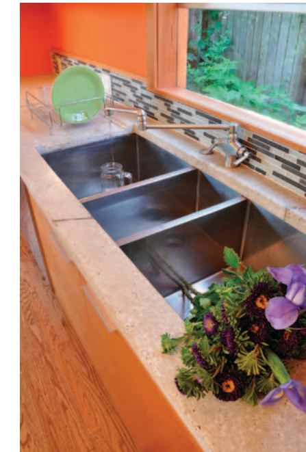
Triple sink. A deep stainless-steel sink sits beneath an articulating faucet and a custom concrete countertop with integrated drain board. The sink has three compartments for maximum utility, with one bowl directing gray water into the garden.
