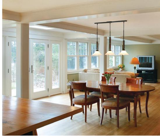
wall by 6 ft. and replaced it with a 16-in. LVL beam supported by two 3½-in.-sq. columns. The beam bisected the ceiling into long, narrow areas disproportionate to one another. I needed to divide the ceiling into sections that made sense visually while incorporating the LVL and columns.
