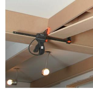
them to the final beam width. To add visual interest to the beams, I use a ¼ in. roundover bit to create a quirked bead at the edges.
