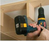
**Long runs go up in sections.** I build and install a full 8-ft. section first, then build the remaining section to fit. The doubled-up ribs at adjoining ends become the backing for the side's joints. Each blocking section is glued to the ceiling with construction adhesive, then screwed into ceiling joists and furring strips that I installed beforehand. For each joist, I use two screws long enough so that at least 1 in. sinks into the joists or furring.
