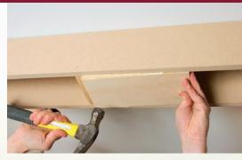
Add blocking no matter where this joint lands. In most finish-carpentry jobs, staggering the joints is a good rule to follow. When running the beam bottoms, I start with a full 8-ft. run as I did with the blocking assembly and sides. But I make sure the joint lands on the other end of the beam. Even if the joint falls on or near a rib, I install extra blocking for a larger nailing surface.
