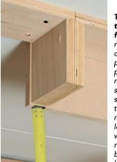
Test-fits reduce the proliferation of four-letter words. | rip the sides based on the ceiling's low point. With the side piece in place, I then measure up from the stringline to make sure the board is the right width to maintain a straight, level run. When I'm working alone, a cleat nailed to the cross beam provides a helping hand.
